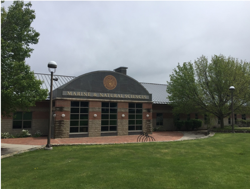
The Marine and Natural Sciences building, Roger Williams University, location for AQUAVET® II classes
