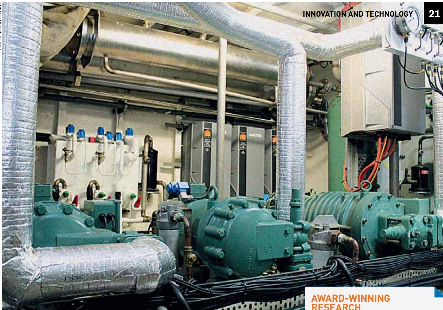
The refitted plant room on board the Gulf Bounty uses R-404A as its refrigerant, replacing R-22.
