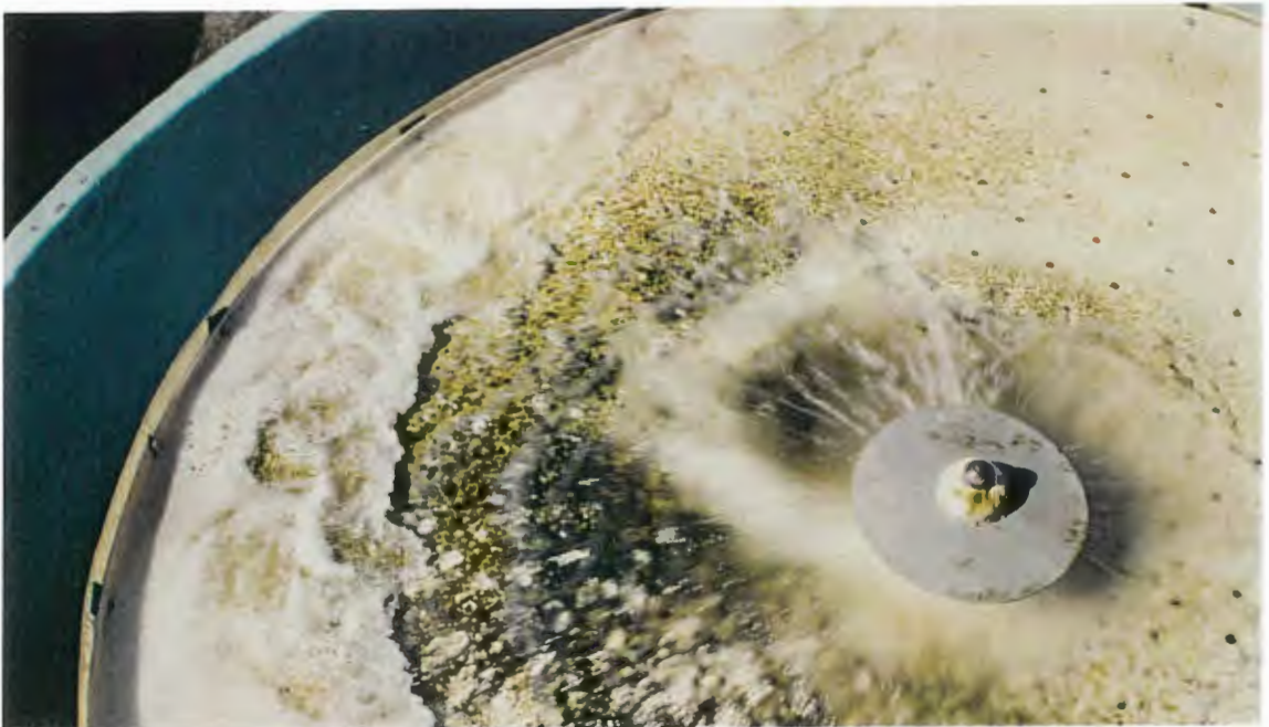
Figure 22 (Above) Examples of the different types of plastic filter media used in biofilters. (Below) Spreader plate on a trickle type biofilter used in a 20,000-litre recirculating system at Northern Fisheries Centre, Cairns. Media used is 80% plastic media ('biocubes') and 20% coral gravel. Water is pumped in at the top of the filter, trickles through the biofilter, and is drained from the bottom of the tank. The perforated spreader plate at the top of the filter ensures that water is spread evenly throughout the entire filter. This particular recirculating system also uses a sand filter for mechanical filtration of particulates, and a foam fractionator.
