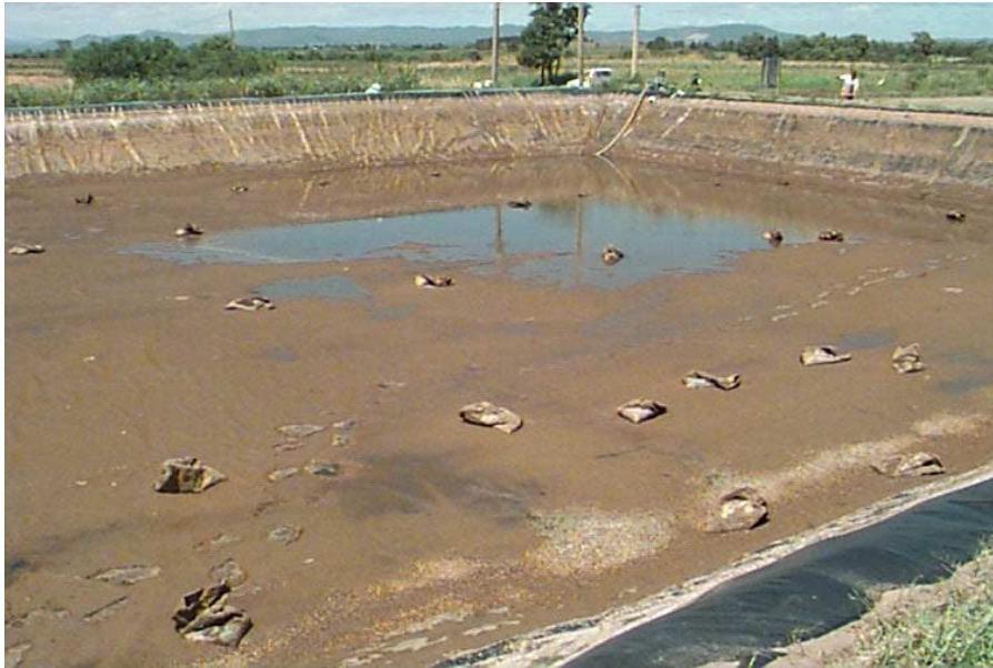
Figure 9. Gold Coast Marine Prawn Farm pilot sedimentation pond, drained after 6 weeks of operation (objects scattered on pond floor are sandbags to weight the pond lining before filling).
