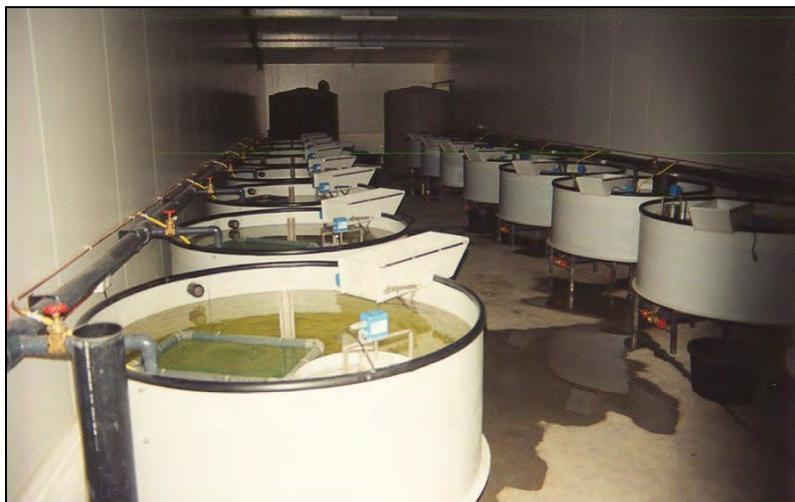
**Fig. 3.1** 1,600 l tanks at Australian Aquaculture Products, which were part of a *Hesy* recirculation system used in the commercial grow-out trial of eels
