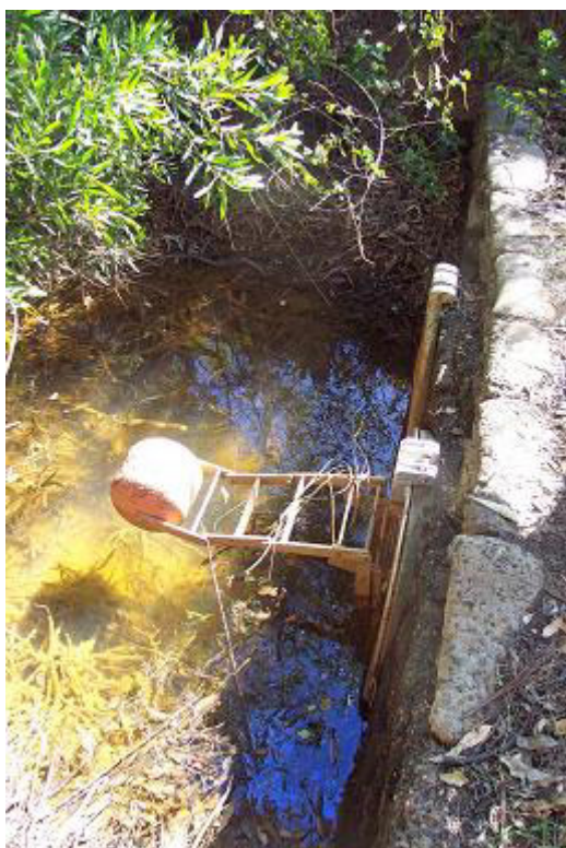
Figure A5.3. Tide-actuated floodgate at Rossglen Drain.
