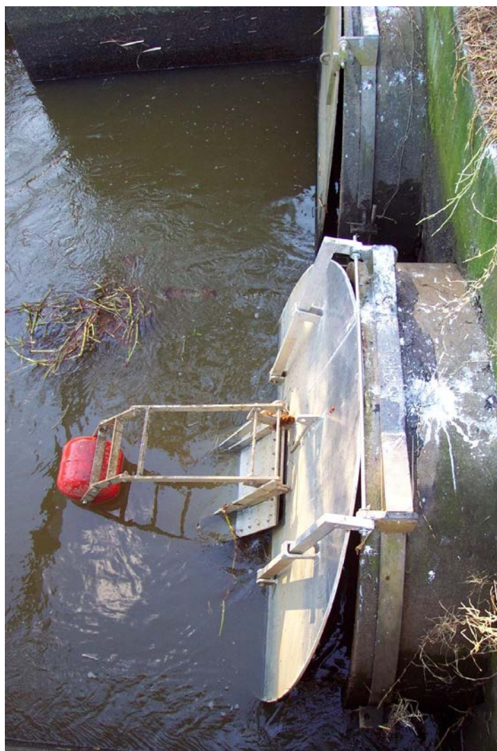
Figure A5.8. Differences in opening size during an outflow between a standard steel floodgate and an aluminium gate fitted with a tide-actuated internal gate.
