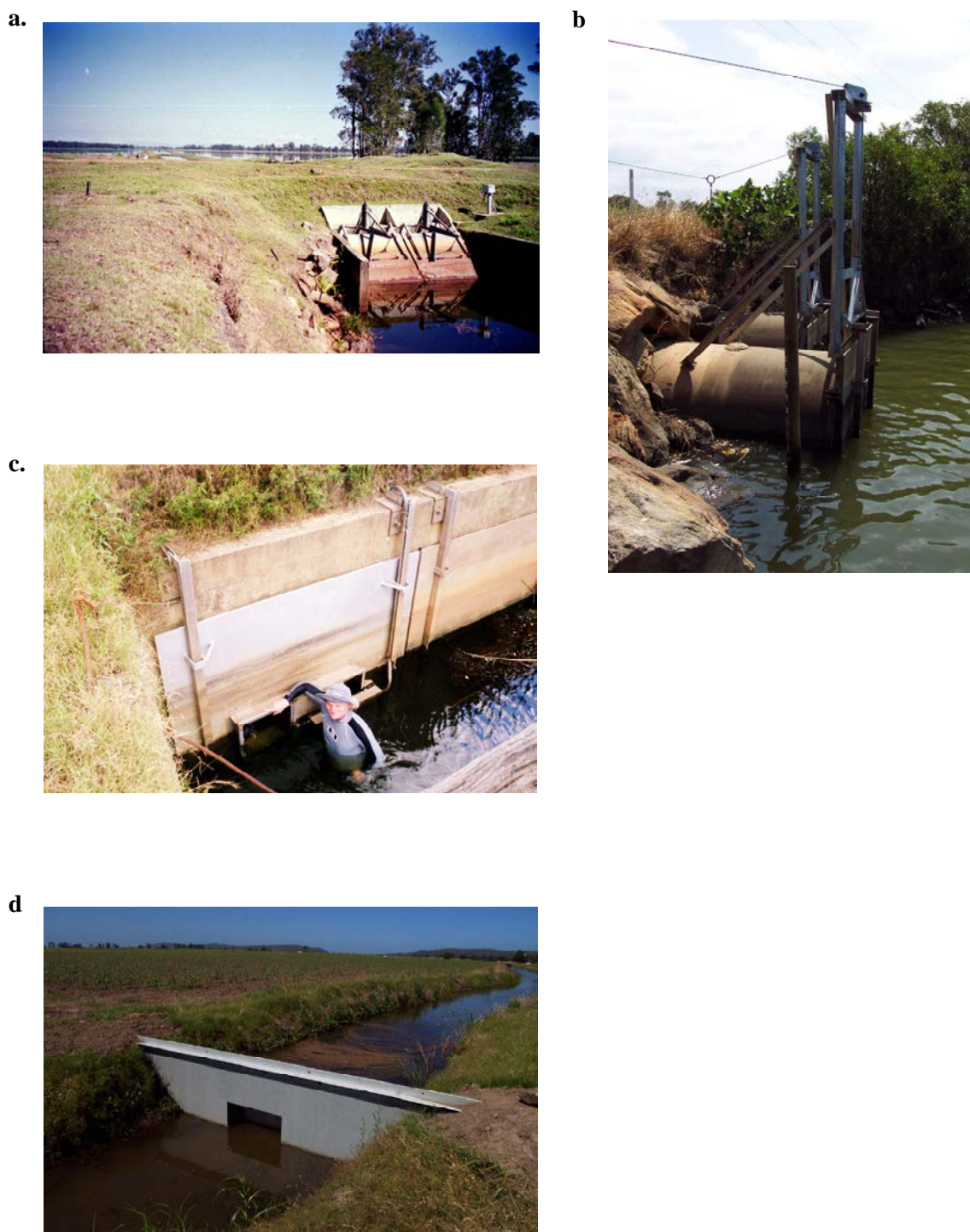
Figure 4.2. Floodgate openings and opening structures in the Clarence river floodplain; a. Wants Drain floodgates in open position, b. vertical liftgate on Marshes Drain, c. mini-sluicgate on Dennys Gully, and d. backwater retention structure in Dennys Gully. Note flooded grazing land on both sides of Wants Drain.
