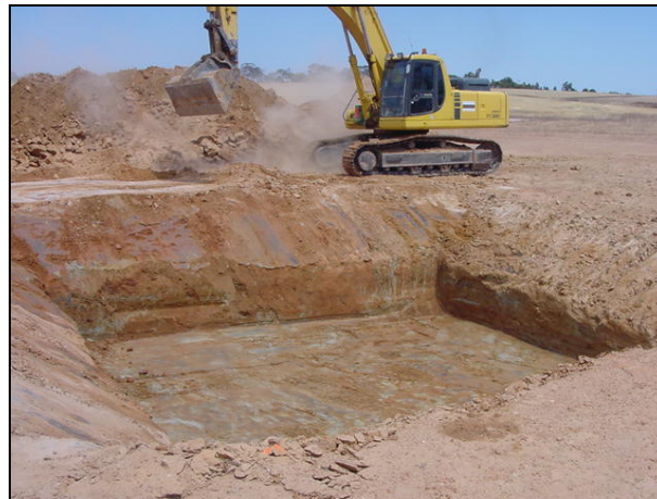
Figure 1. Excavation of a 100m 2 research pond at Northam showing wall batters.
