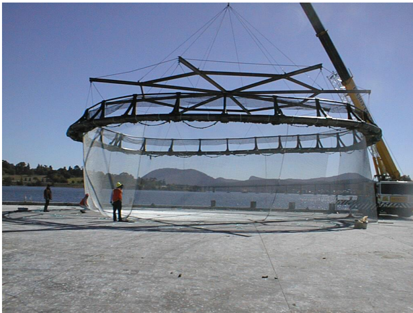
Figure 4 : Onesteel Marinemesh fit-up onto 80m pen at Hobart
