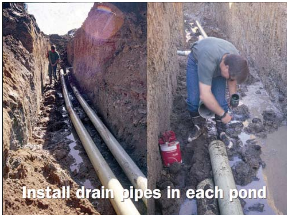
Slide 12. Install drain pipes in each pond.
