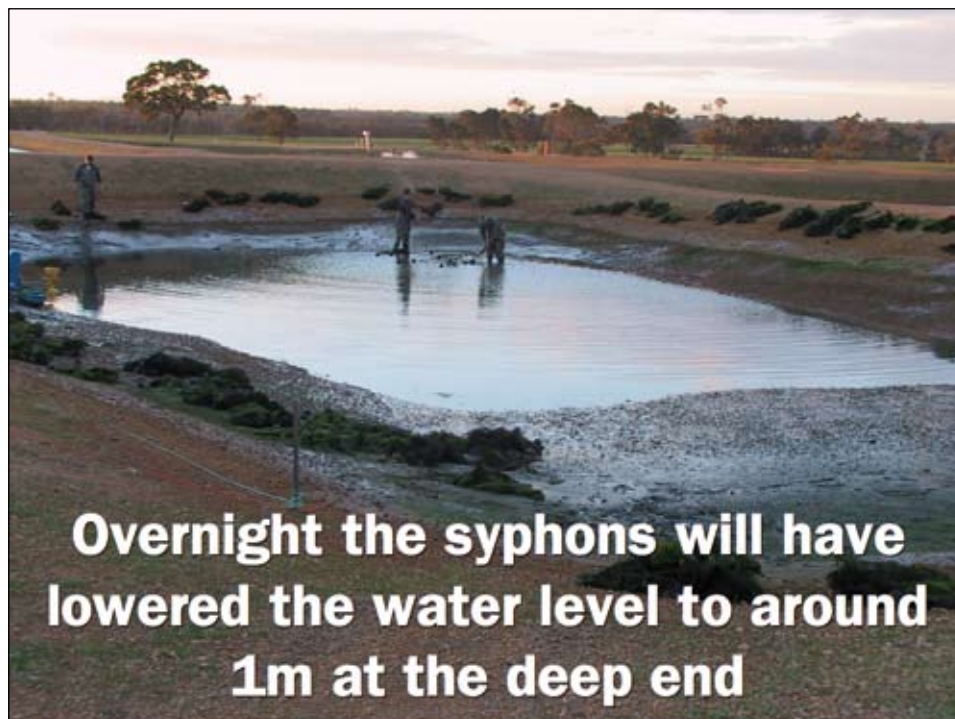
Slide 33. Overnight the syphons will have lowered the water level to around 1m at the deep end.
