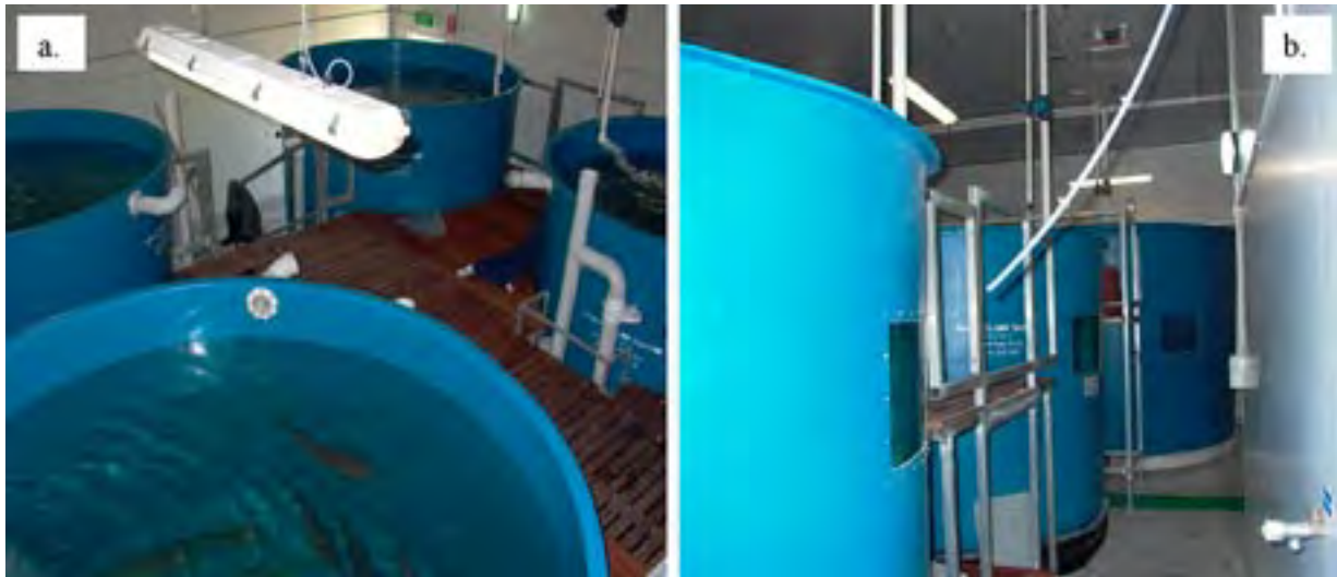
Figure 2 a) Four 10,000L broodstock holding tanks in a controlled environment room within the R&D Hatchery facility at the SAASC. b) Side view of the broodstock tanks, 2 x 10,000L front and centre and a 22,000L tank at rear.
