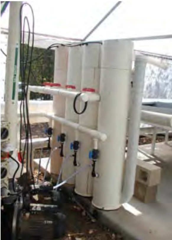
▲ Figure 4. Algal scrubbers are part of the secondary water treatment system.
