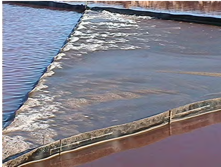
Figure 24. Biomass / cyst collector operating.
