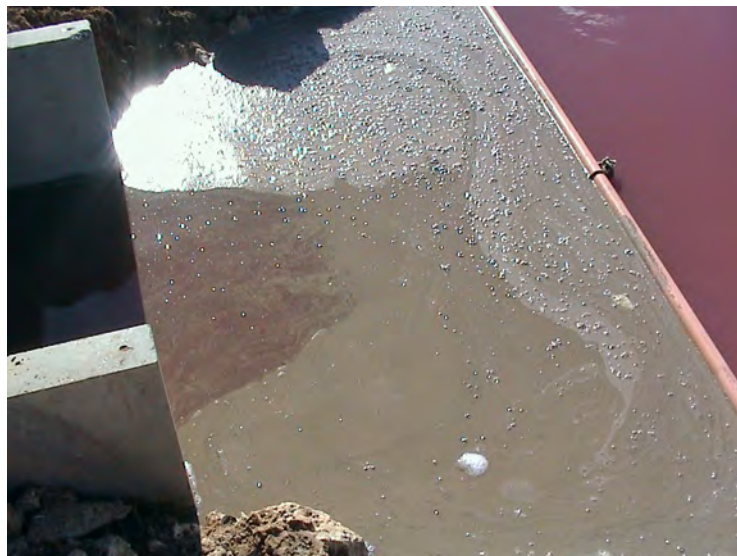
Figure 16. Artemia cysts collected in culverts.
