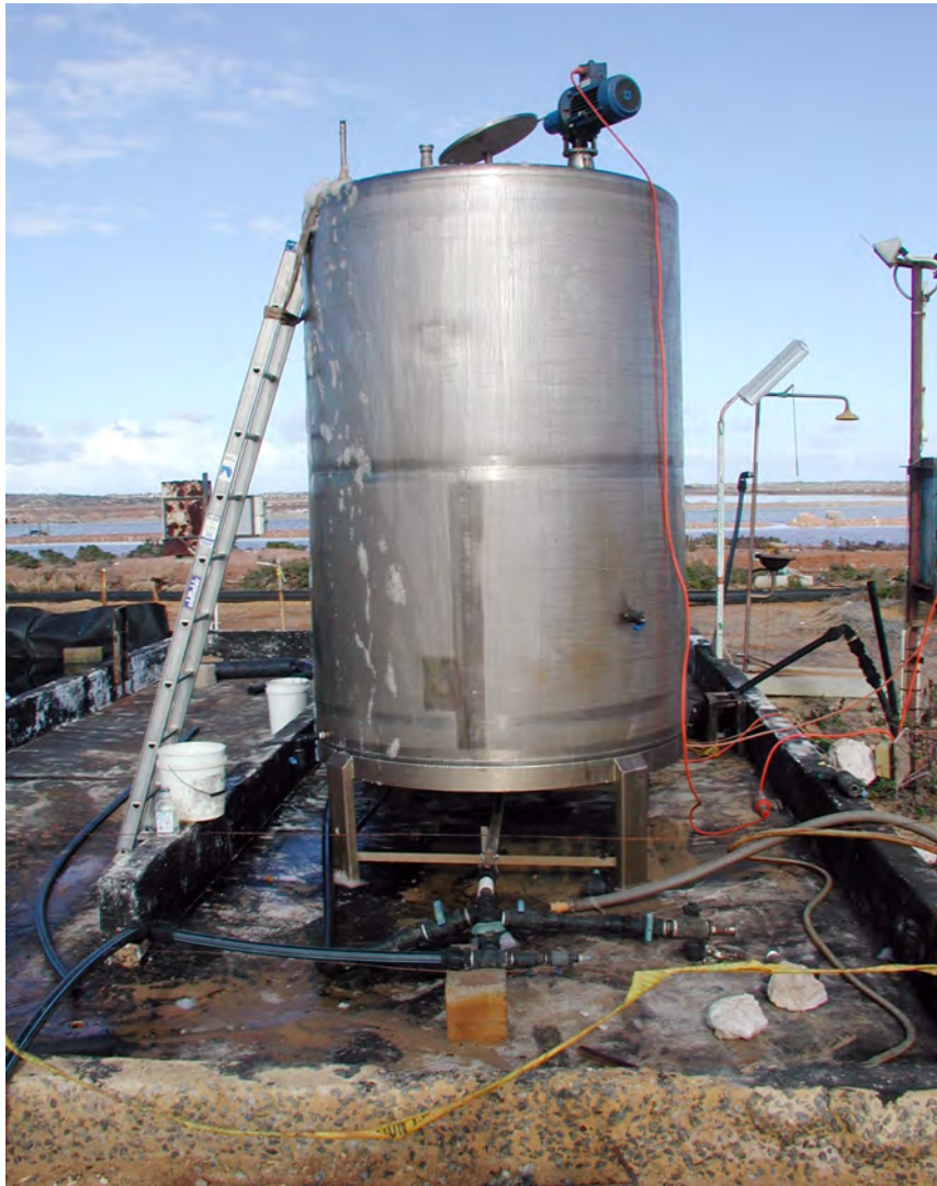
Figure 7. 3,000 l tank used for hatching.
