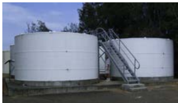
Fibreglass seawater storage tanks
