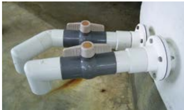
Drain valve apparatus on 20,000 litre larval rearing tank
