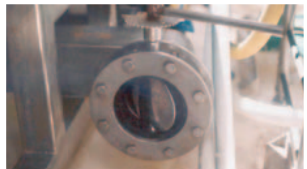
Wafer butterfly valve.
