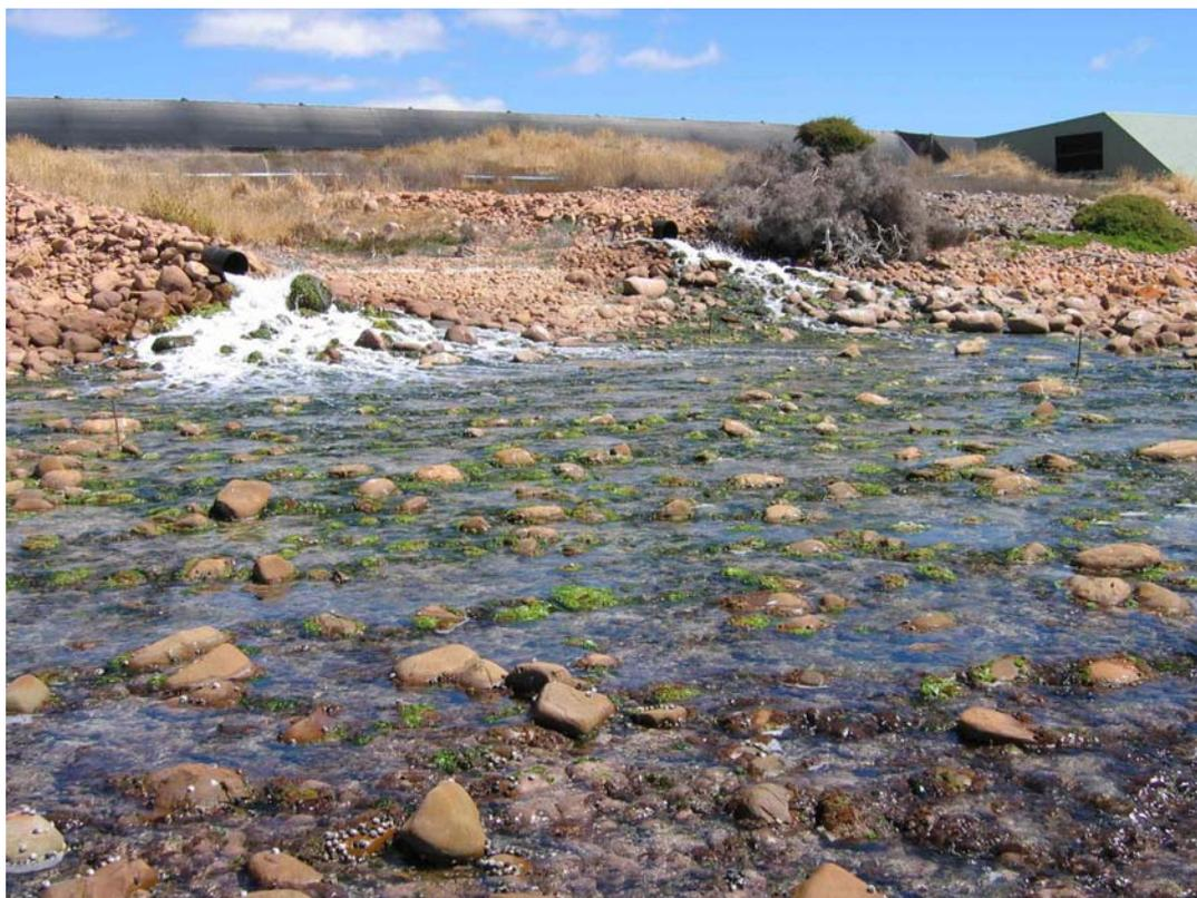
**Figure 4.1.** Outfall pipes discharging land-based abalone farm seawater to the intertidal shoreline at Smith Bay, Kangaroo Island. Note how the outflow of water has essentially transformed the area from an intertidal to a subtidal habitat.
