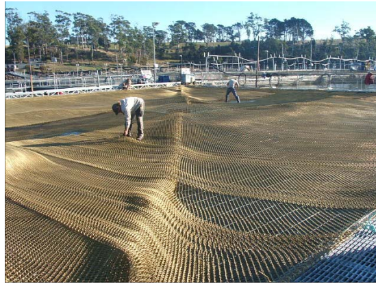
Fig 8.1.3.2.2. The installation of a brass cage to prevent seal predation of salmonids in the Tamar River.
