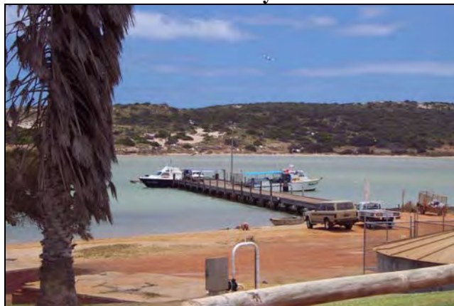
Plate 3: Service Jetty in Kalbarri
