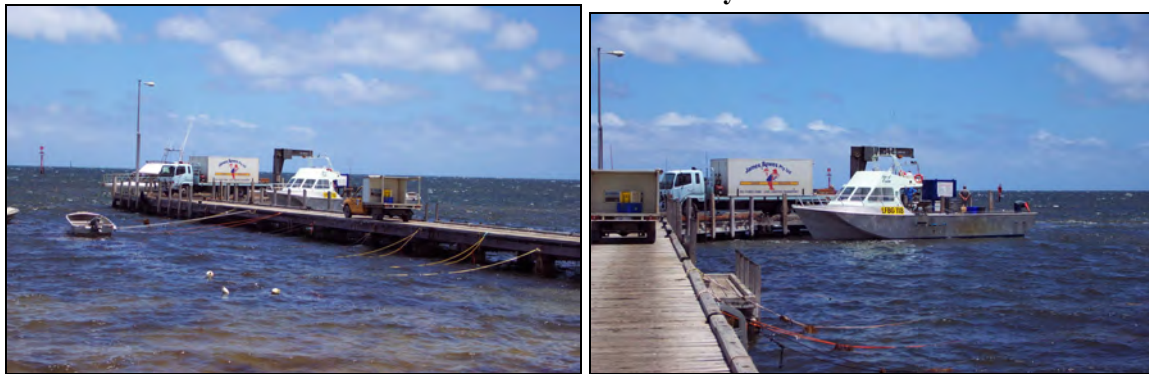
Plates 1A and 1B: Timber Jetty in Leeman
