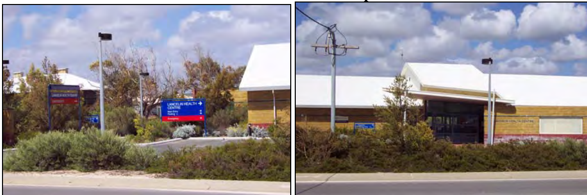
Plates 5A and 5B: Lancelin Multi-Purpose Health Centre
