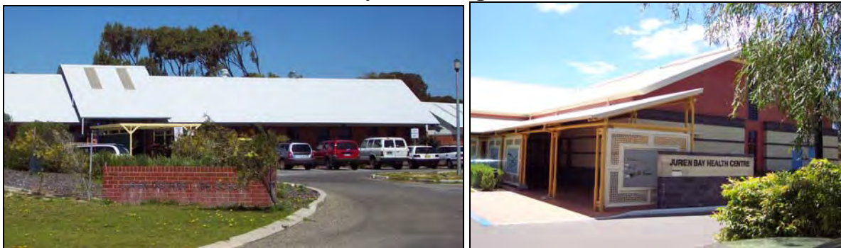
Plates 9A and 9B: Jurien Bay District High School and Health Centre
