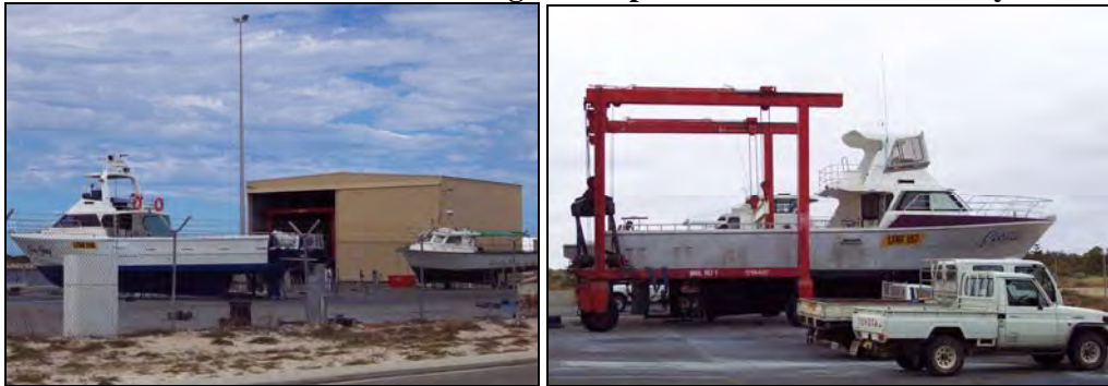
Plates 3A and 3B: Boat-lifting and Repair Facilities in Jurien Bay
