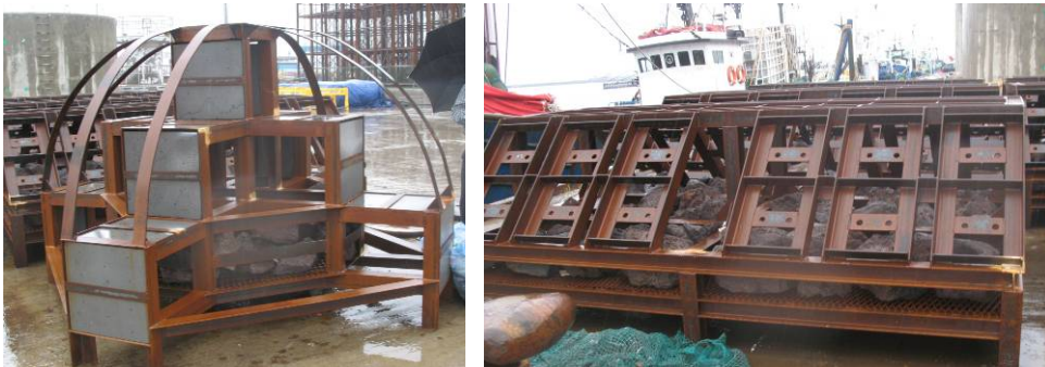
Complex steel and ceramic plate modules with stone ballast Cheju Do Korea
