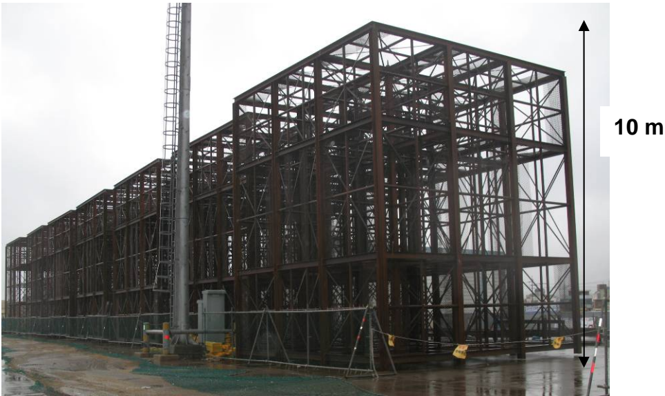
Complex steel reef module for rockfish and pelagic fish Cheju Do, Korea (note complex voids and high vertical relief)
