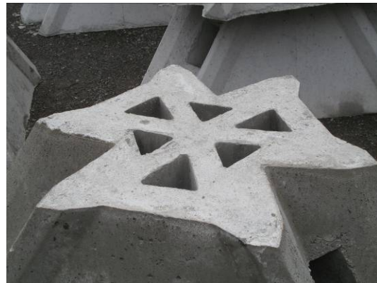
Shellfish void units fit in each corner of tetrahedral modules above. Cheju Do Korea
