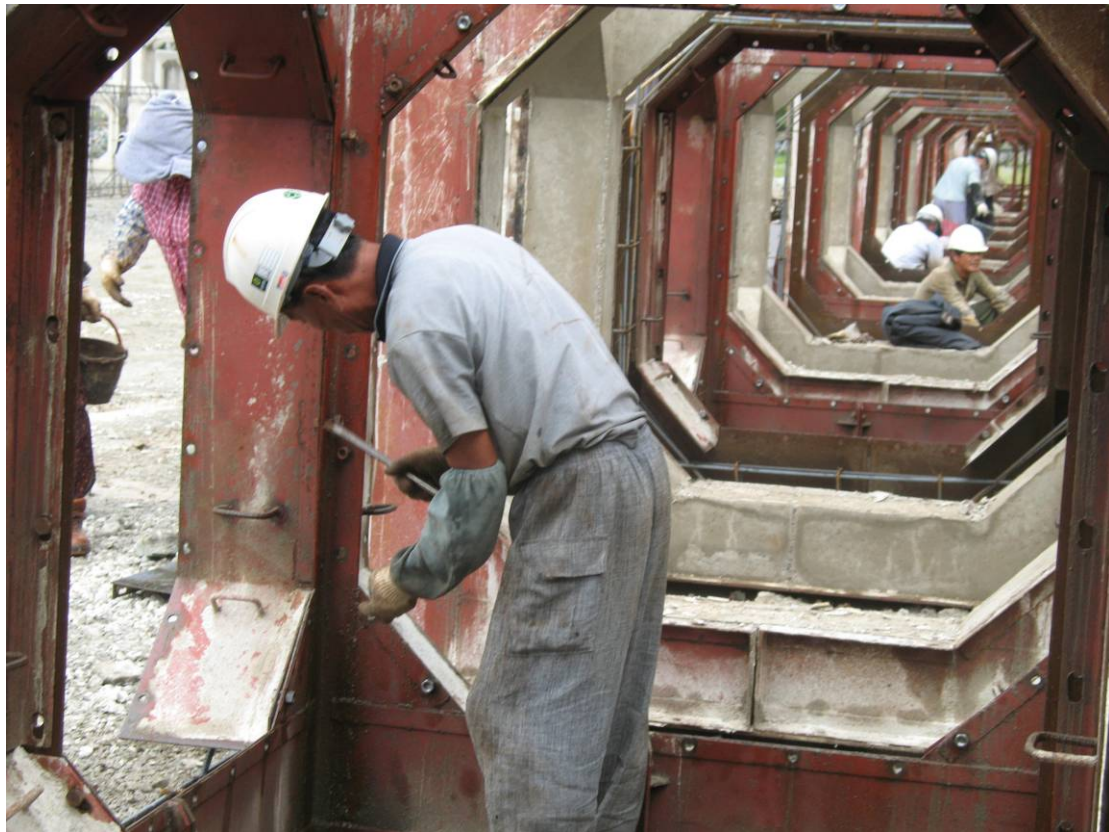
Concrete reef construction detail, Korea
