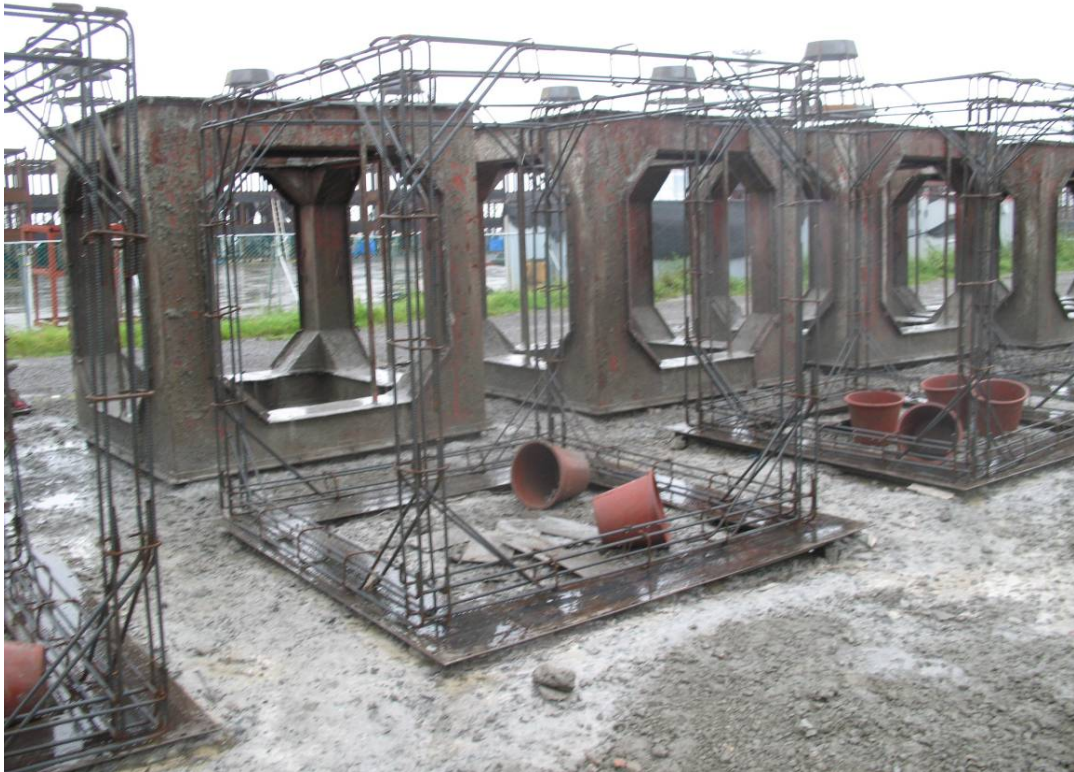
Concrete reef moulds, Korea
