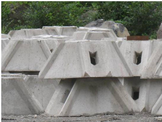
Shellfish void units fit in each corner of tetrahedral modules above. Cheju Do Korea
