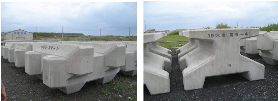
Experimental artificial reef modules for algae and abalone, Sugawara Corp. Nakaminato, Japan
