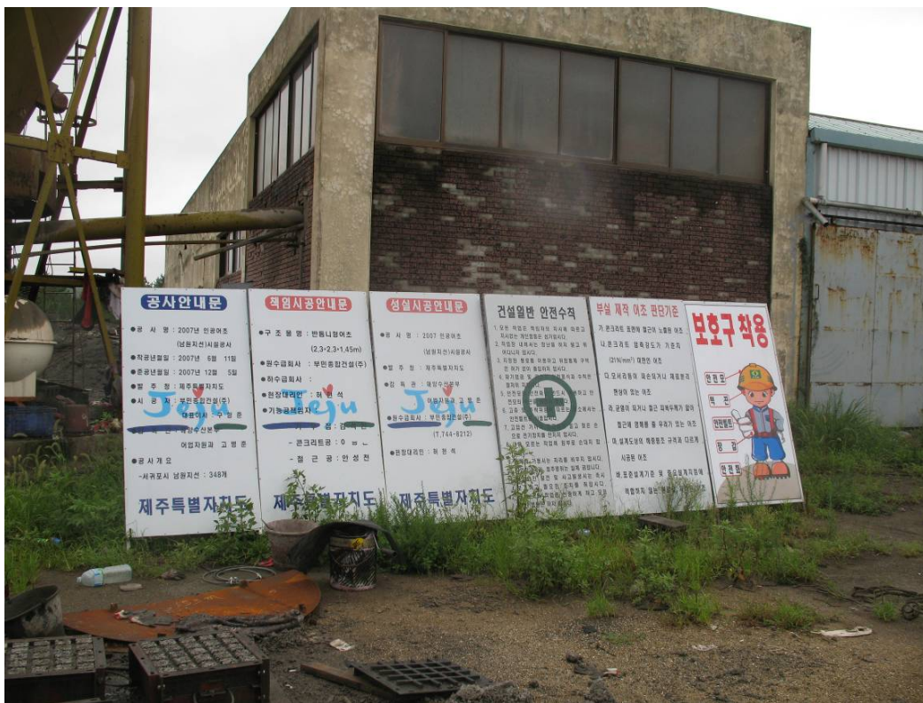
Concrete reef construction, Korea
