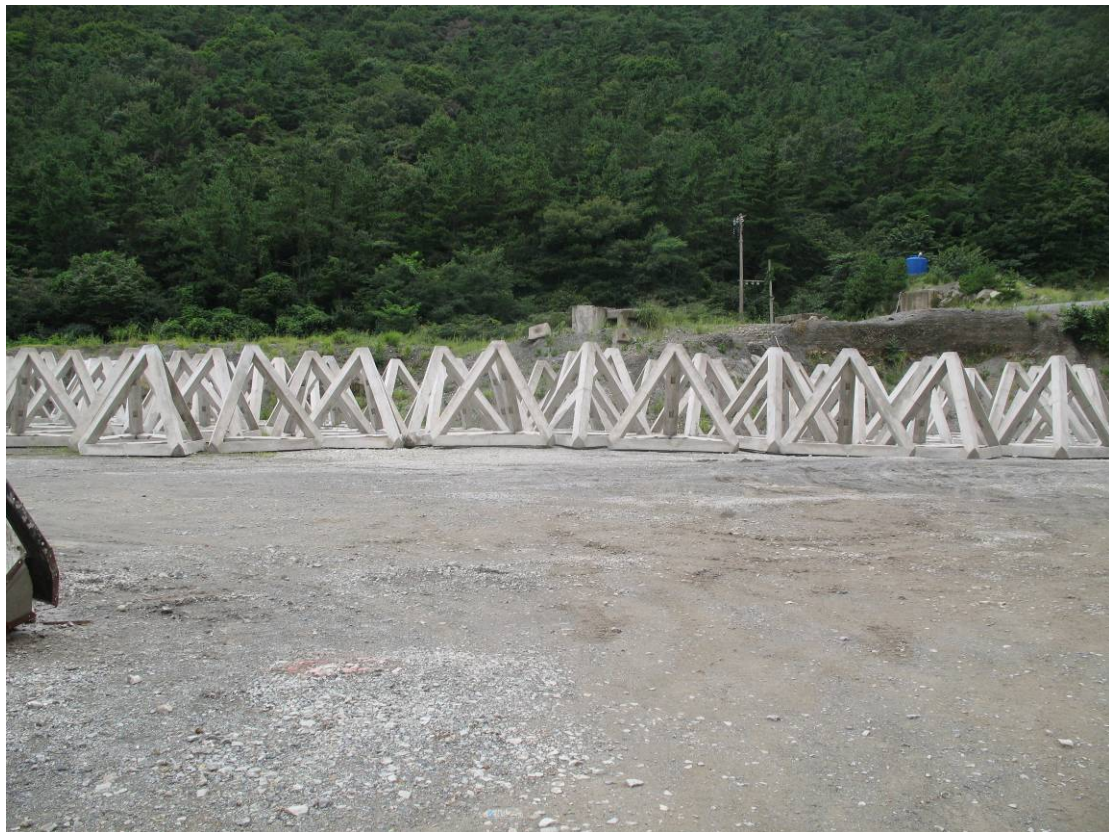
Mixed purpose reef construction, Korea
