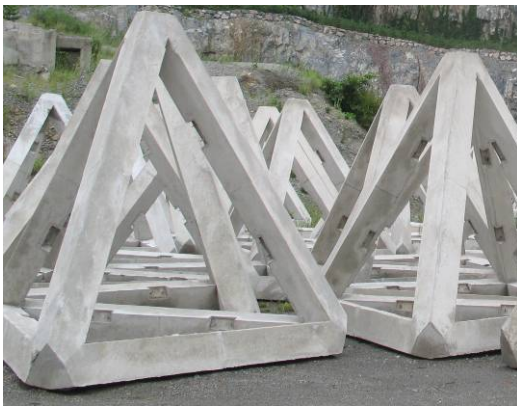
Tetrahedral concrete fish and shellfish modules Cheju Do, Korea
