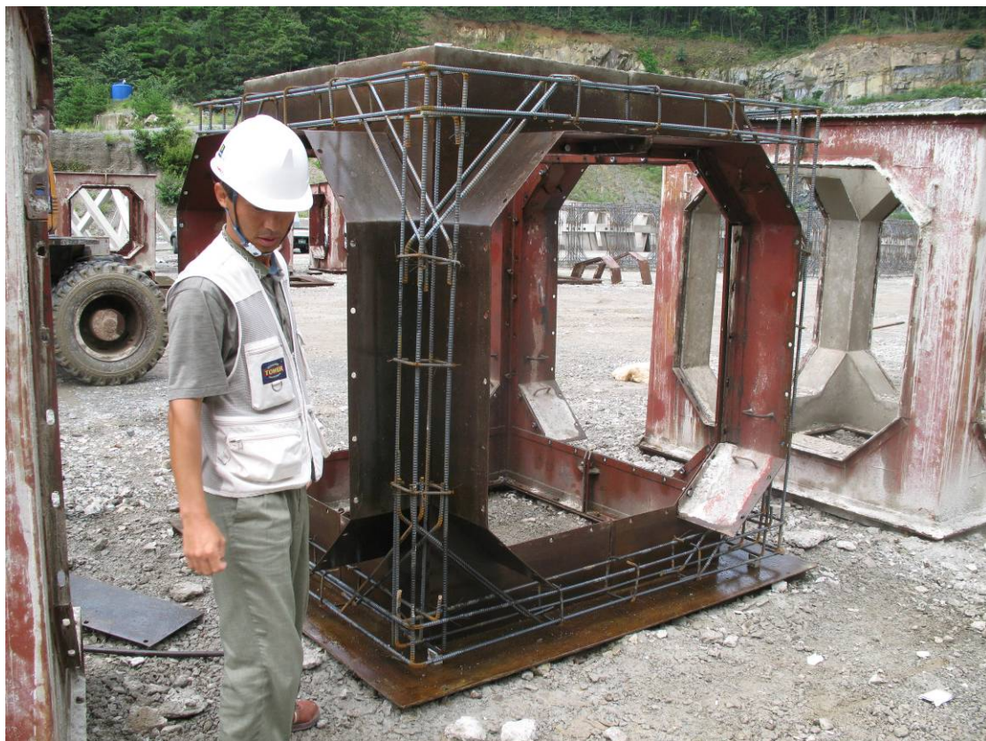
Concrete reef construction detail, Korea
