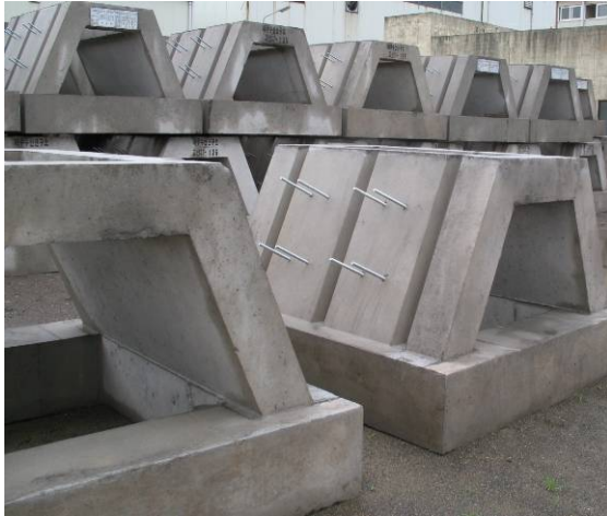
Algae and shellfish concrete reef modules and oyster shell attachment plate Cheju Do, Korea
