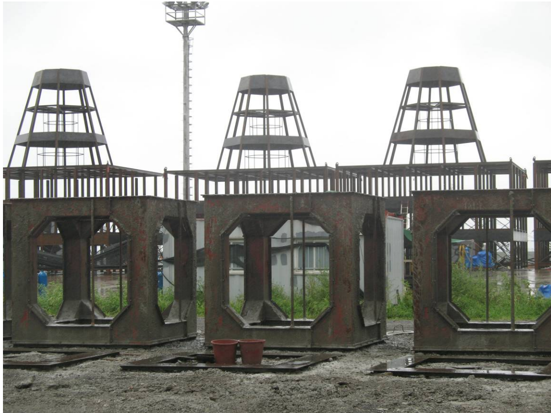
Concrete moulds (fore), Steel reefs (rear), Korea
