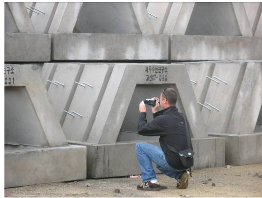
Oyster shell aggregate module for algae and top shell Cheju Do, Korea
