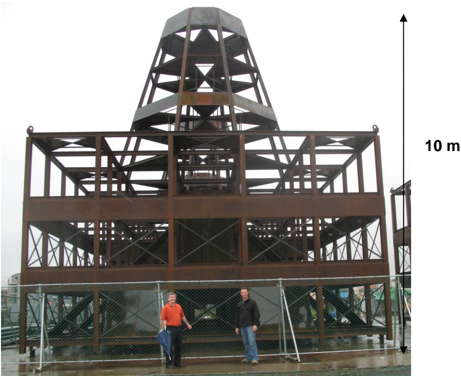
Steel reef module for pelagic and demersal fish Cheju Do Korea (note lower panels to deflect current up through the structure)
