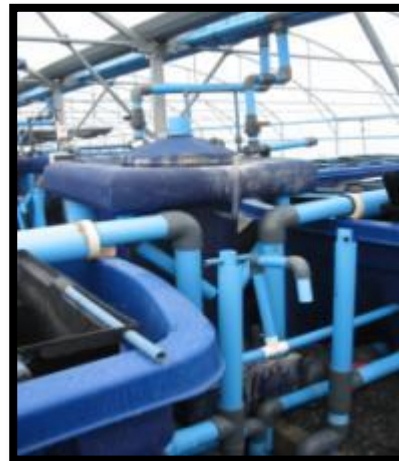
Figure 19: Abalone grow-out airlift system
