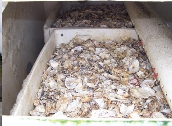
Wet storage oyster shell biofilter
