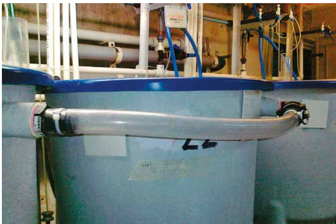
Figure 22. Double tank system for passive transfer of larvae
