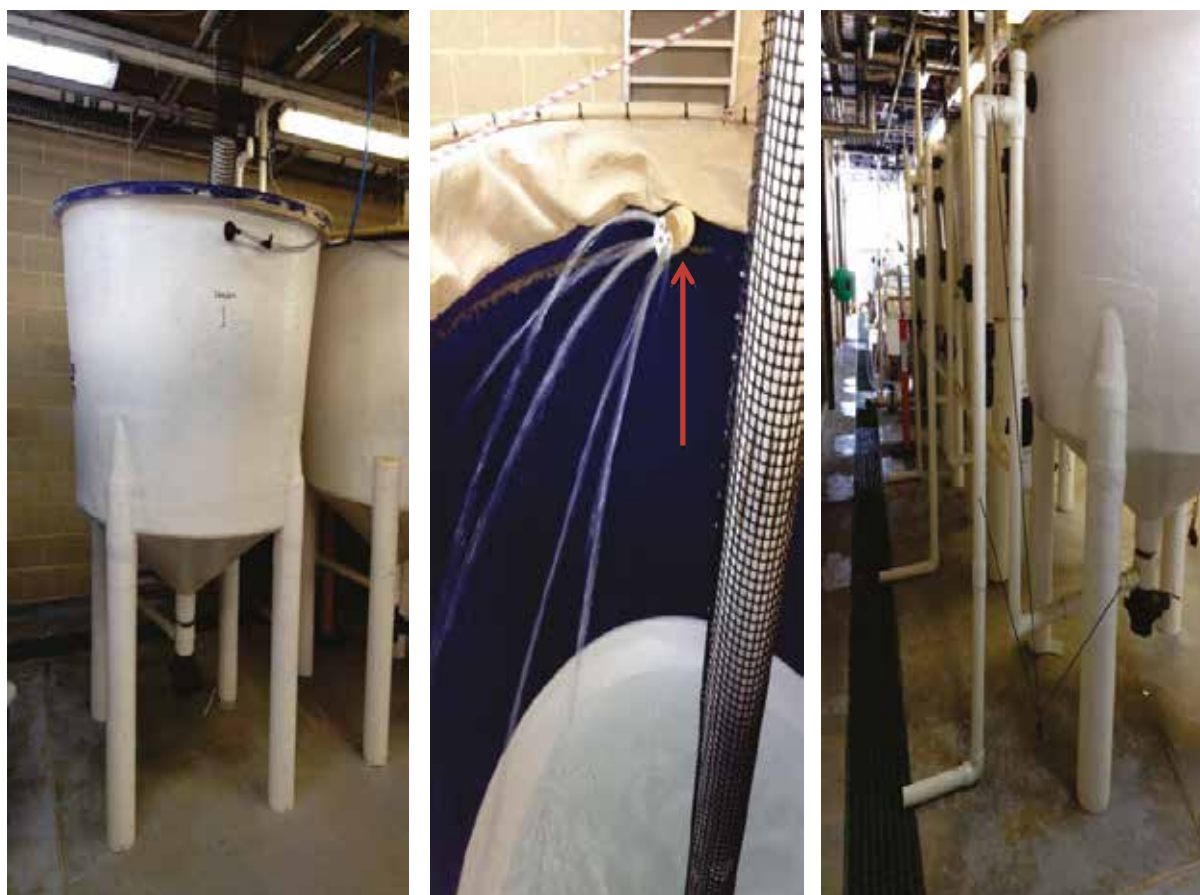
Figure 58. 2300 Lt system and tank components. Red arrow indicates hard plumbed seawater inlet.
