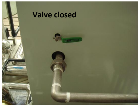
Figure 12. Dryer water reclaim valve in the closed position
