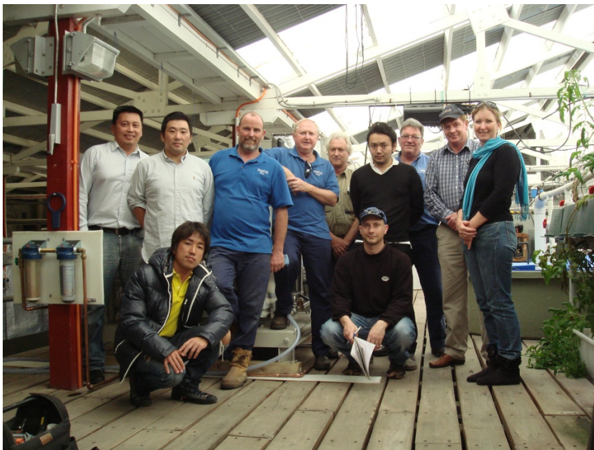
Figure 2: The dryer installation team. Inventor Dr Fukimoto is standing second from left.
