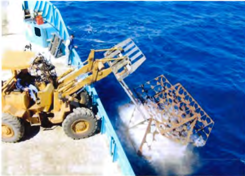
Materials of opportunity dumped at Roy Rufus artificial reef Hervey Bay Queensland (Photo courtesy of Bundaberg and Districts Artificial Reef Association)
