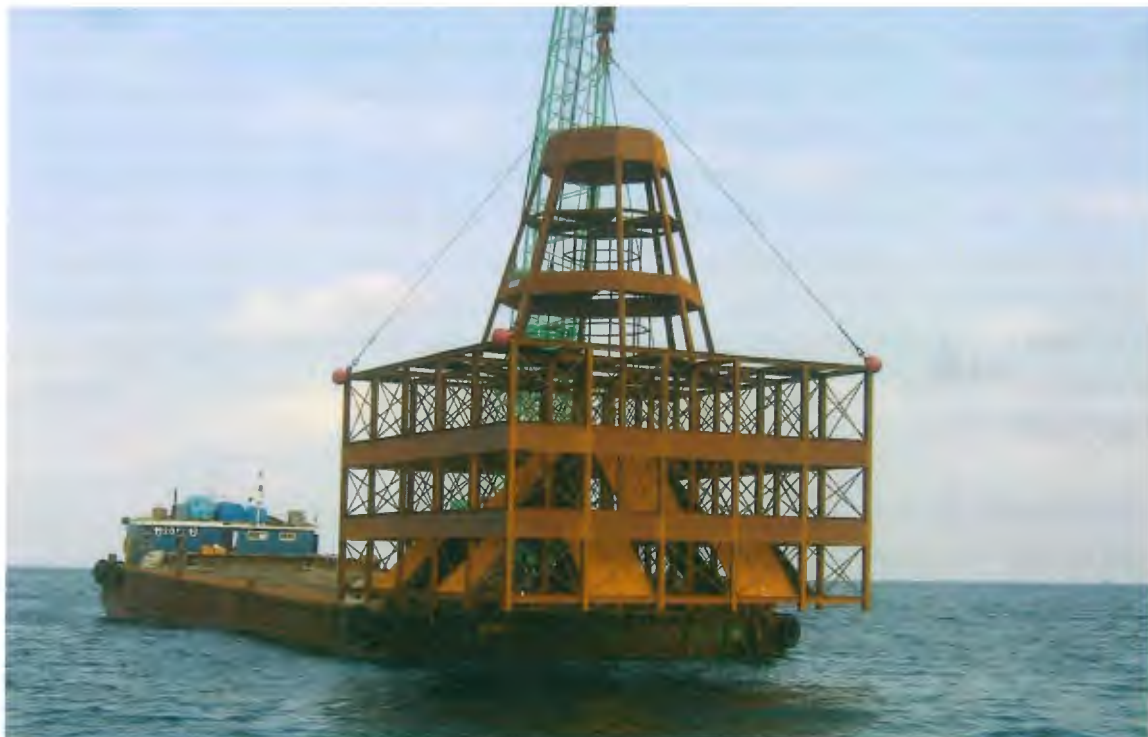
Korean steel artificial reef module
