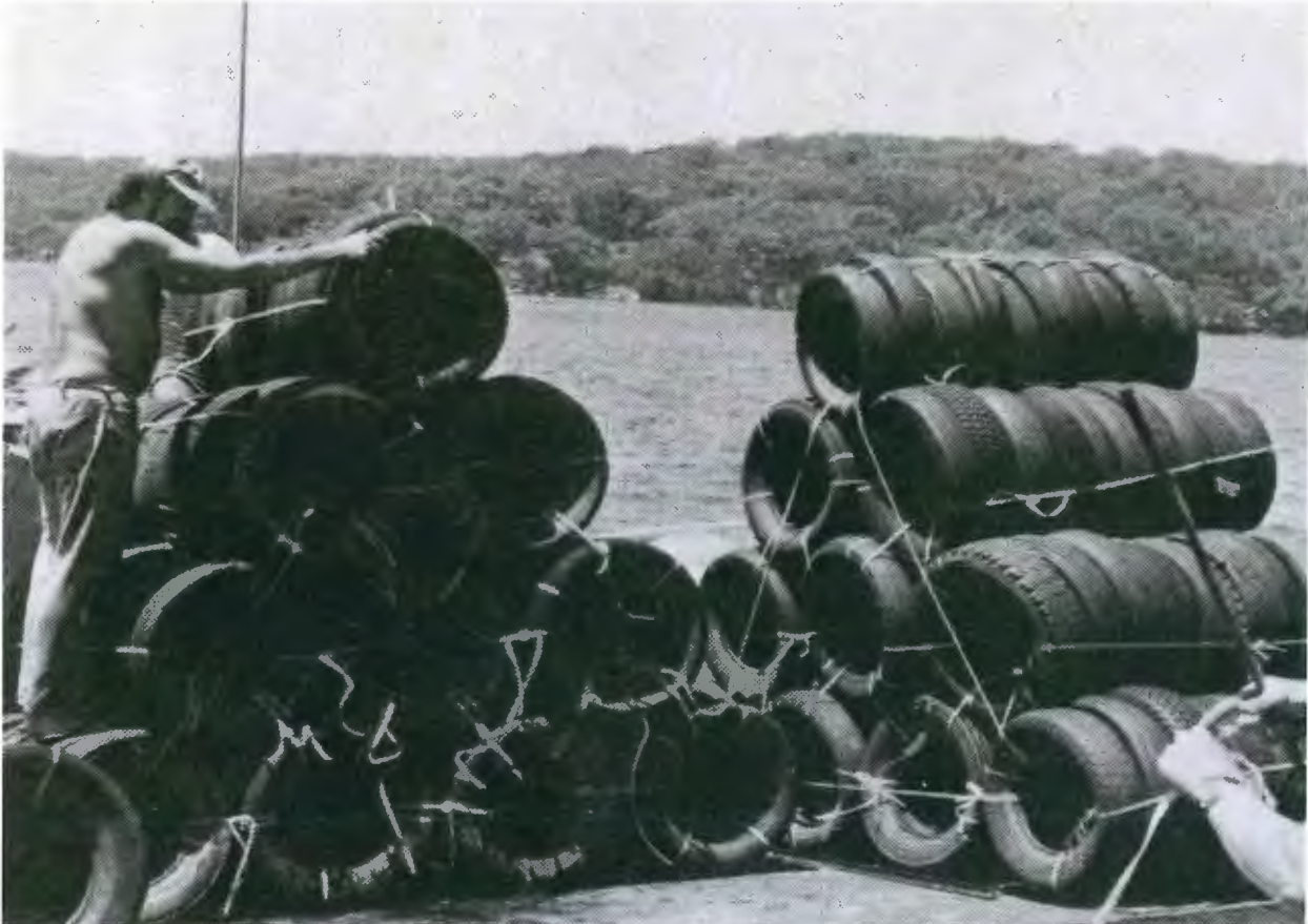
Tyre modules assembled for deployment in Lake Macquarie NSW
