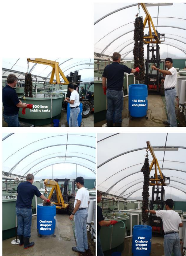
Figure 13: Onshore thermal treatment of the mussel droppers
