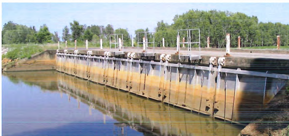
Floodgates prevent fish from accessing former wetland 'grow-out' areas further upstream.
