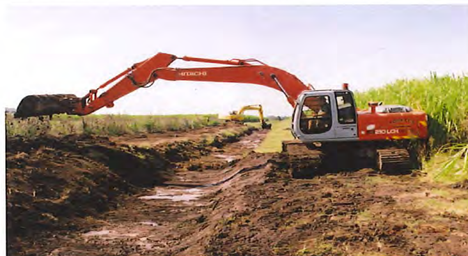
Excavators are used to re-shape or completely fill in drains
