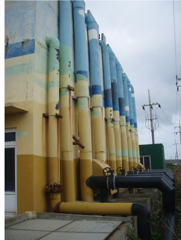
Image – Sand filter and header tank, pump ashore, Flounder farm (win Win Seafood Corp), Jeju Island
