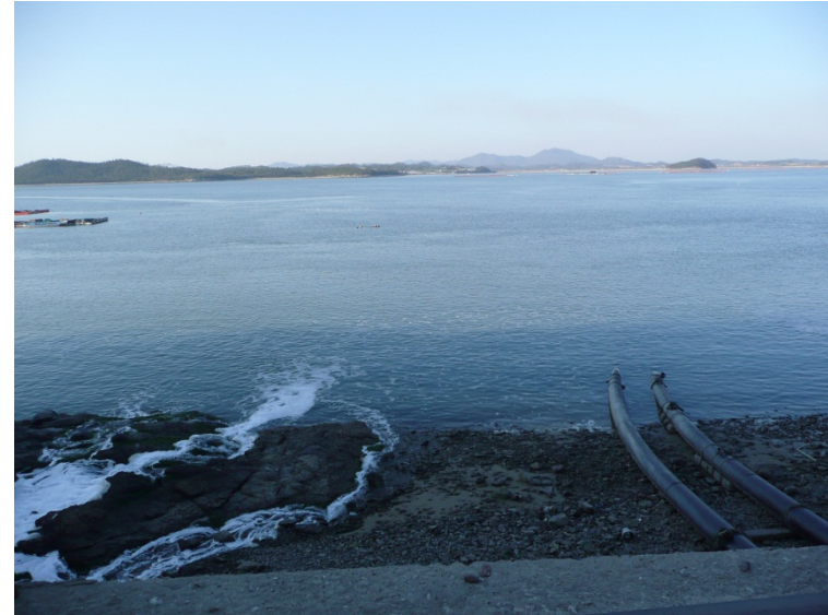
Image – water intake and discharge , Abalone Nursery, Jindo
