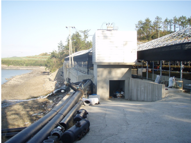
Image – pump shed and water discharge , Abalone Nursery, Jindo
