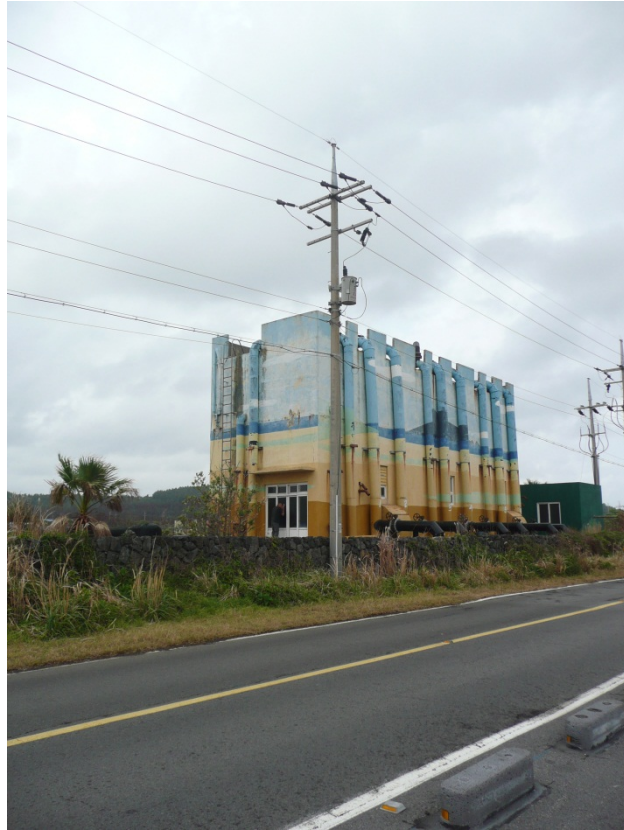
Image – Sand filter and header tank, pump ashore, Flounder farm (win Win Seafood Corp), Jeju Island
