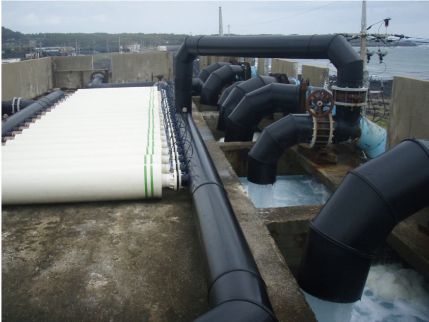
Image – Sand filter and header tank, pump ashore, Flounder farm (win Win Seafood Corp), Jeju Island
