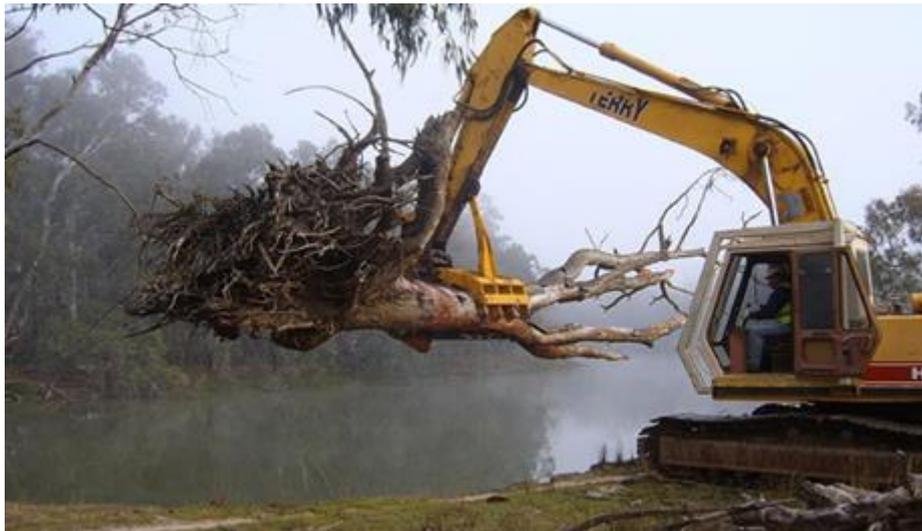
**Figure 68:** Large snag being installed on the Murray River (Source: Fish Habitat Network).
