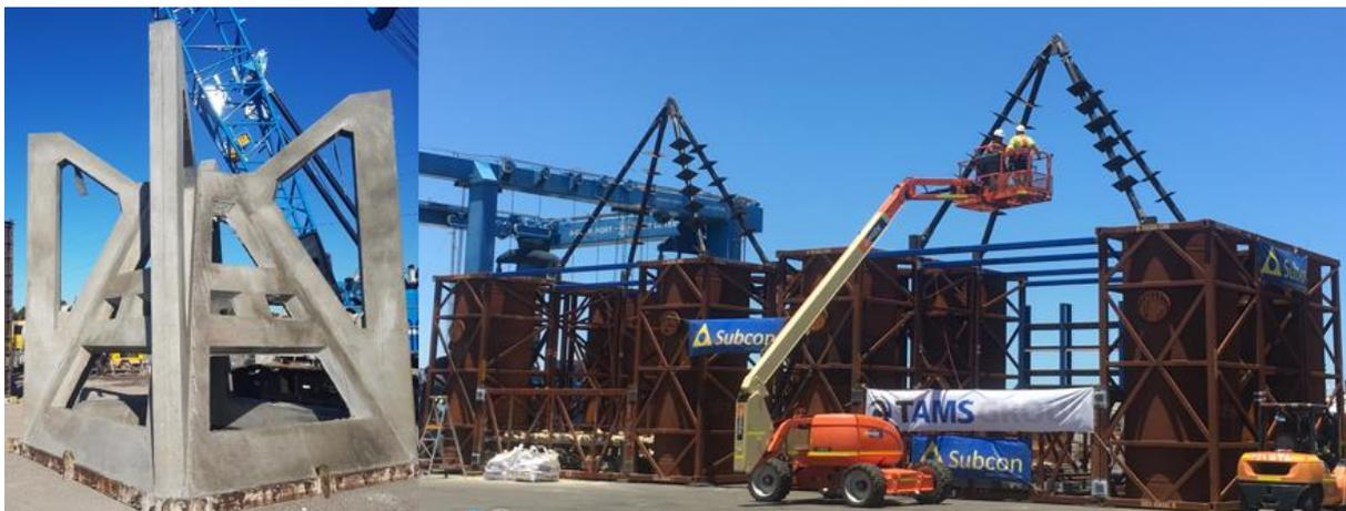
**Figure 19:** Reef Pyramid<sup>TM</sup> (left) and Fish Towers<sup>TM</sup> (right), steel modules constructed and deployed by Subcon (Recfishwest).
