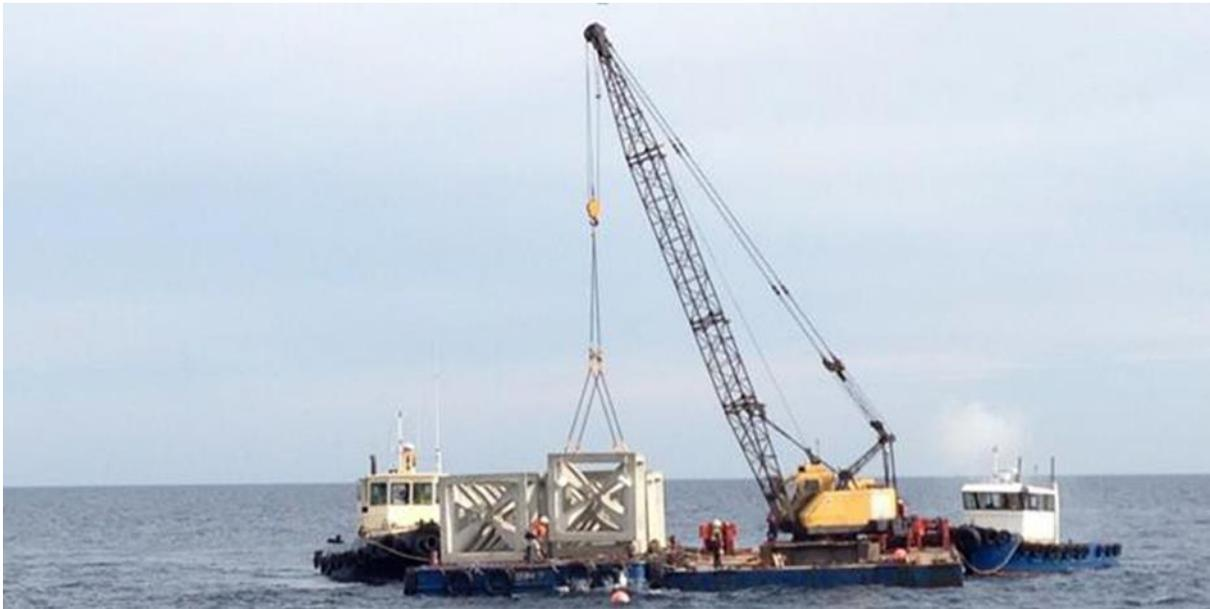
**Figure 66:** Crane and barge deployment of concrete artificial reef modules in Western Australia.
