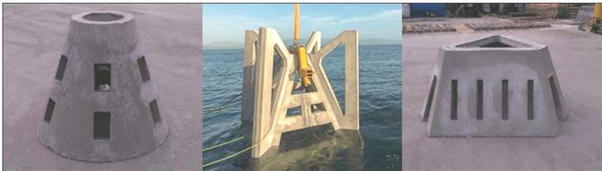
**Figure 60:** Different concrete artificial reef module designs for different purposes and target species (<http://www.subcon.com/>).
