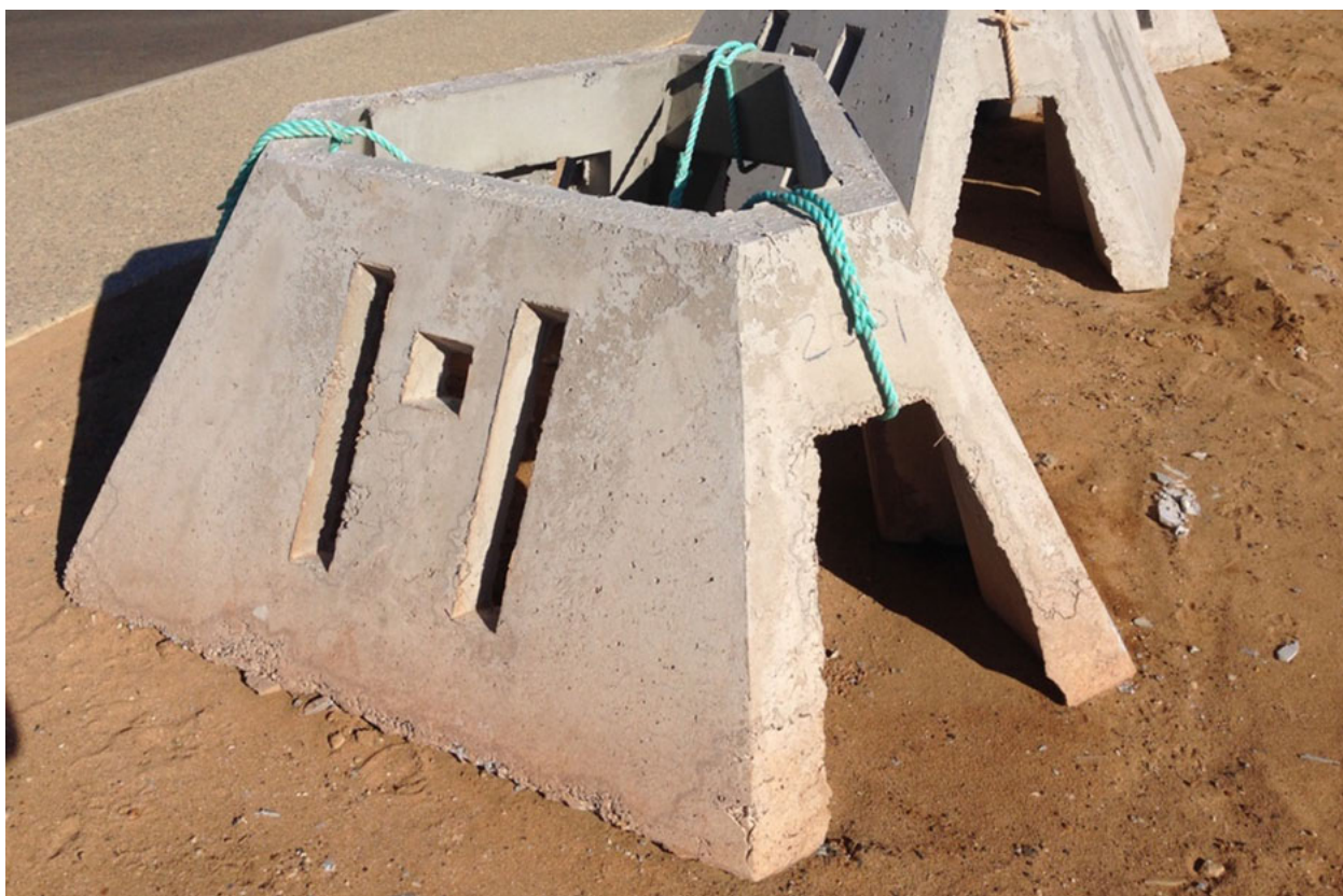
Figure 3.2 An artificial habitat constructed by OGA. The design prevents sand submergence, traps algae, provides shelter for seeded juvenile abalone and contains sufficient surface area for colonisation
