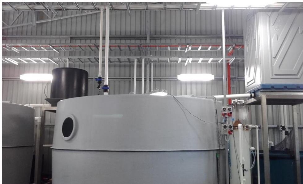
Figure 23. Thirty (30) m 3 RAS tanks at PSFI for nursery culture of juvenile YTK. RAS 1 (with black MBBR filter) and RAS 2 (with Biogill® filter). Note a foam fractionator below Biogill® of RAS 2.
