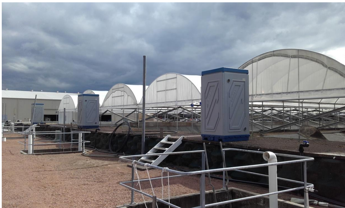
Figure 24. Four, 250m 3 plastic-lined ponds covered with polyhouse at PSFI with Biogill® installed for water quality management.
