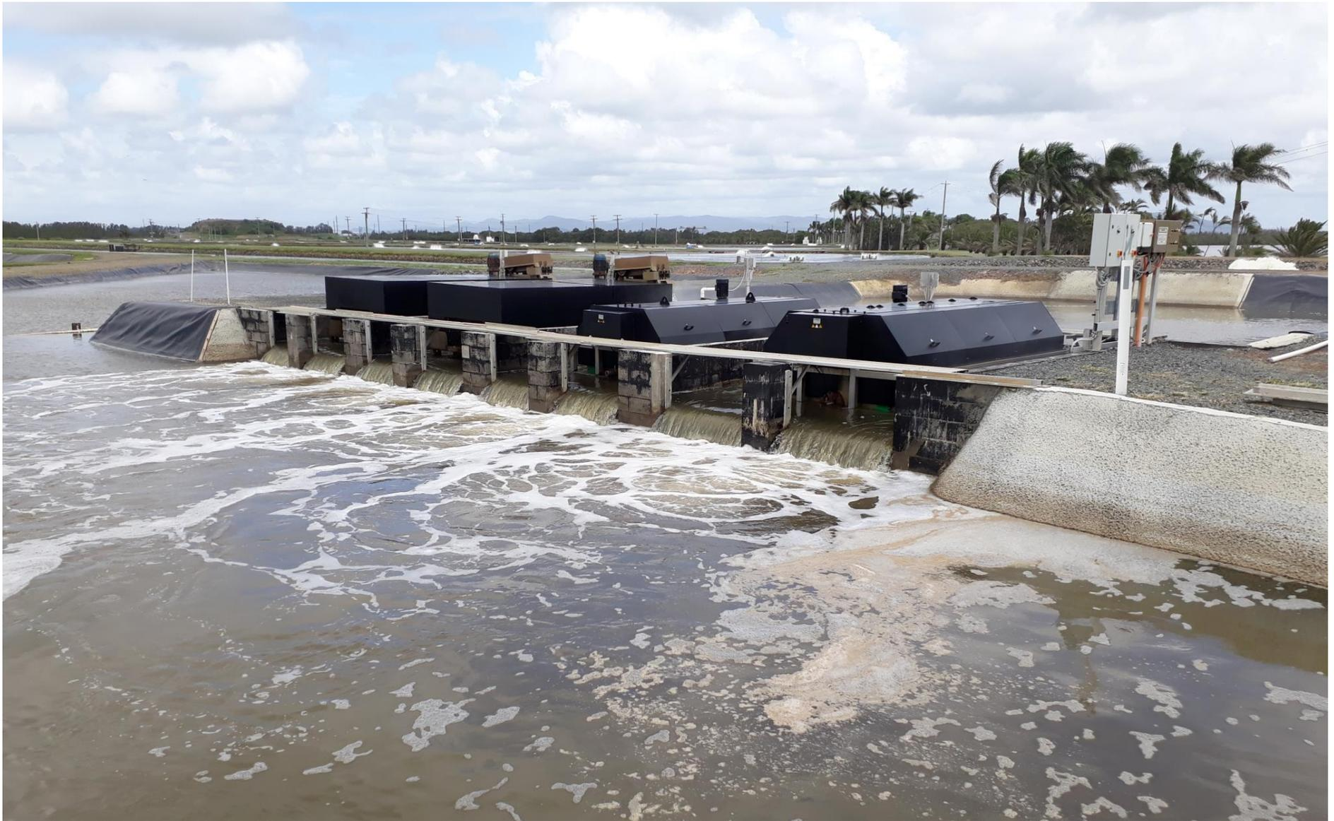
*Figure 4. Sampling of potential WSSV vectors was undertaken at various locations (including pre and post drum filter) around the inlet canals of the three operational prawn farms on the Logan River in late April and early May 2020. A range of biosecurity measures had been implemented since 2016-17, including installation of drum filters, which at this farm (Farm C) can filter 1200 L of intake water per second (4320 m<sup>3</sup>/hr) to a nominal 50 microns.*
