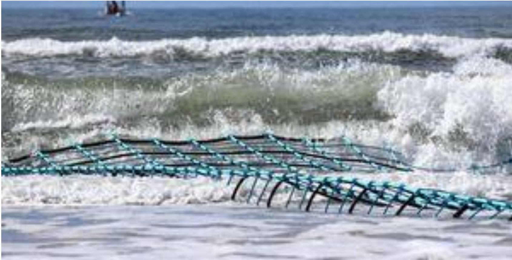
Shark Barrier Fail – NSW North Coast
