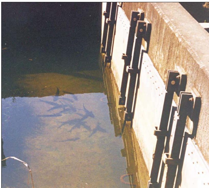
Figure 25. Floodgates act as barriers to fish and can restrict their access to upstream habitat areas.
