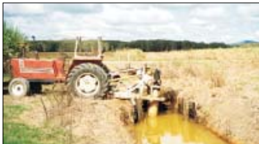
Figure 12. In low-lying areas drains are sometimes pumped to assist water removal. Lowering drain water levels by pumping in ASS areas which have high soil permeability can increase drain water acidity and enhance acid export (see Figure 31).
